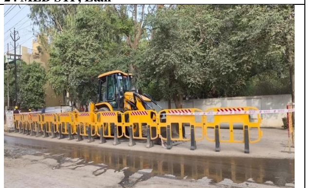
Sewer Laying, Mirzapur
